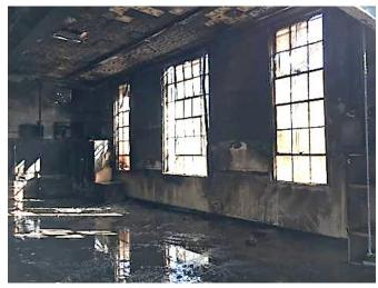
Recently, an electrical fire resulted in the total loss of multiple classroom bungalows at one of our schools. The fire was caused by overloaded electrical outlets. Extension cords were also connected in series to a surge protector. This combination of illegal and unsafe practices overloaded the circuit. Fortunately, no one was injured during the fire, but the cost of repairs is substantial, and the loss of classroom space is a true hardship.
